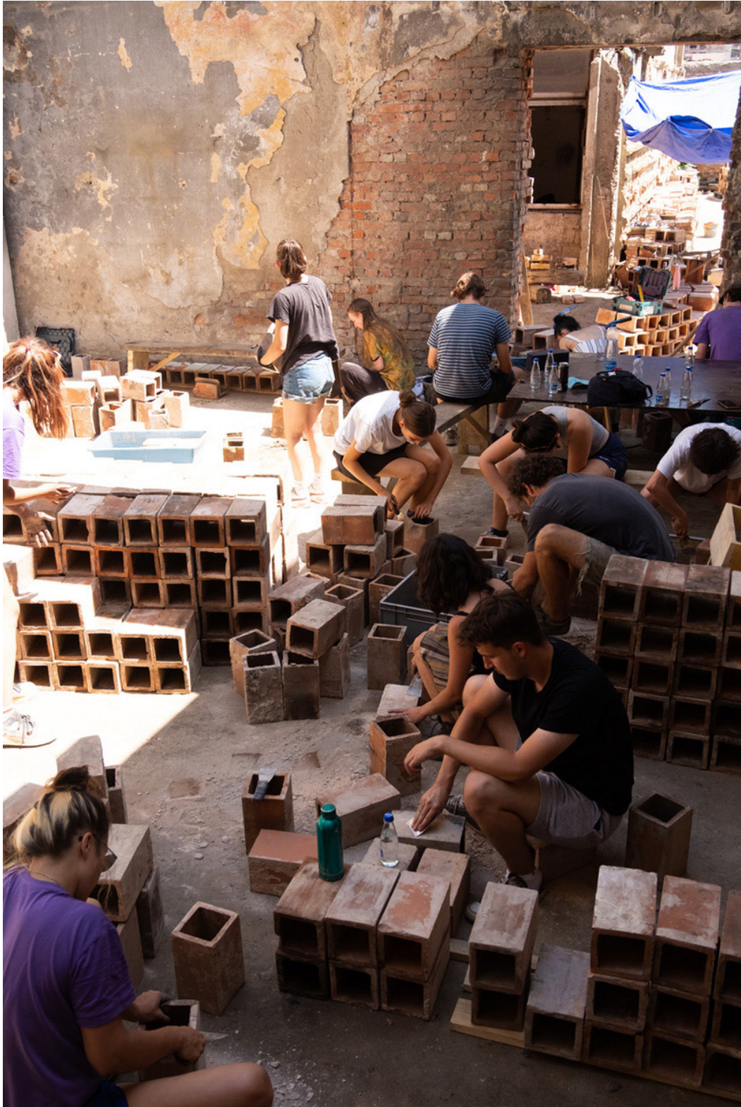
raumlaborberlin, (Working on) Common Ground, 2022 Pristina, Kosovo
